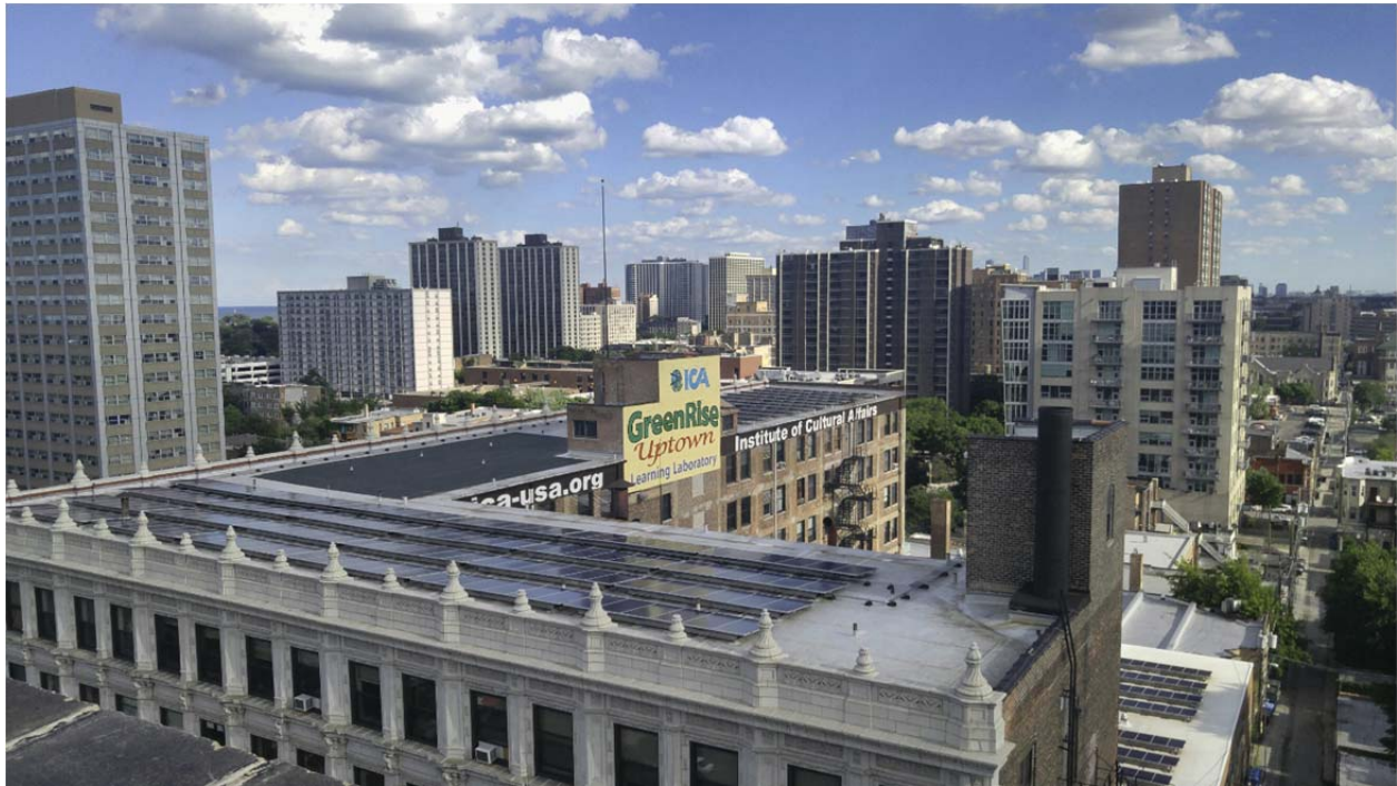
ROOFTOP SOLAR ARRAY
